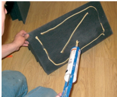
Applying adhesive to a foam bass-trap.
