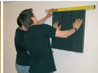
A spirit level will help to keep things looking neat.
